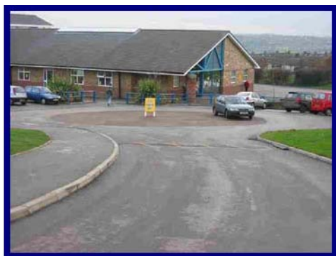
Staff car parking in front of school
